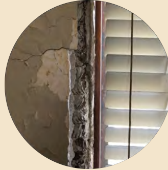
The building INTERIOR shows signs of excessive water damage
